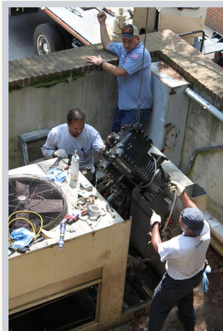
*A little less than a year after a direct lightning strike to the chiller caused compressor failure in our HVAC system, an electrical surge after another storm fried the compressor for a second time in the summer of 2014. Upgrading the HVAC system is a top priority in the 2014-2019 Strategic Plan.*
